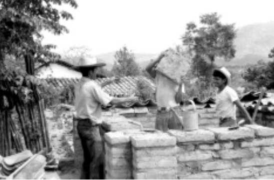
Working and learning together how to build correctly to prevent damage.
