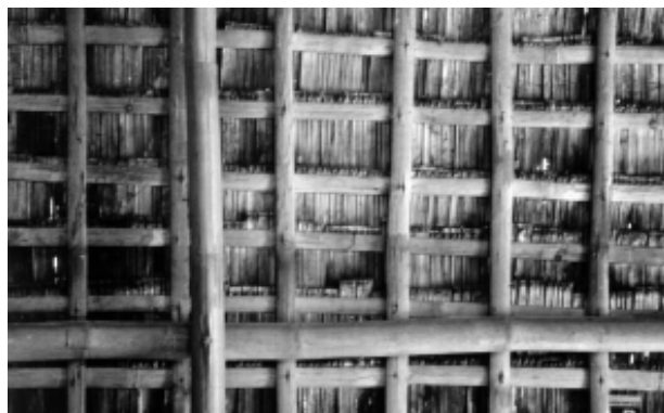
Inside view of a split bamboo tile roof
