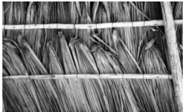
Inside view of fan-shaped palm thatch
