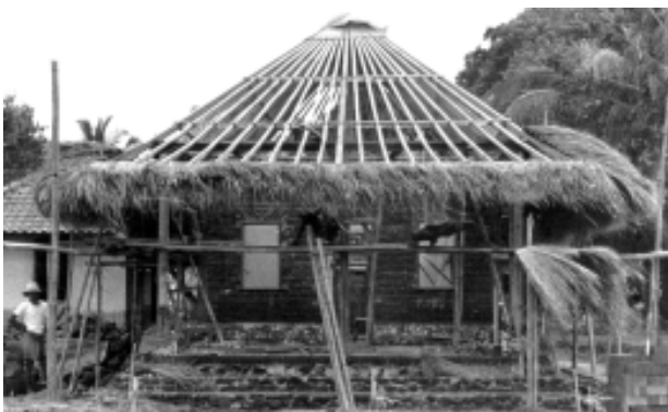
in Indonesia this type of palm thatch is up to 200mm thick
