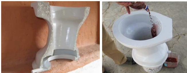
Fig. 4: Cross section of urine diversion bowl (left) where urine collects in the little trough at the bottom as demonstrated in urine diversion bowl (right) (source: CHP, 2009)
