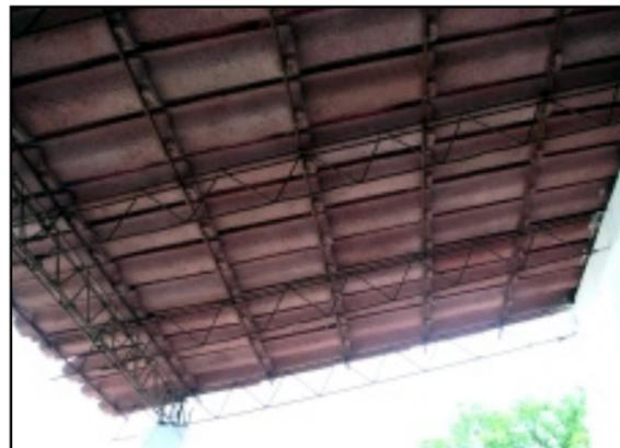
**The picture above shows a bar structure (it is important to highlight that it was made in a factory and is of unusually good quality): The beams are placed at a distance of 75cm and bars of 3/8" are used as battens. These bars deform with the weight of the tiles and the finished roofs is irregular. This solution becomes more expensive than using C-section and tubes.**
