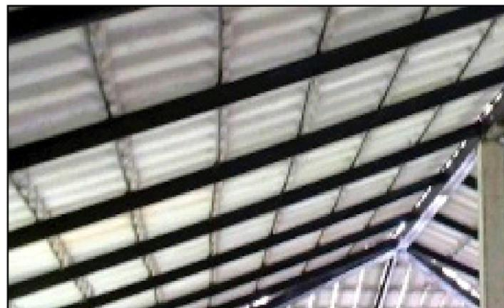
**This picture clearly shows the deficiency of the bar battens. Even on beams of «C-sections», it is difficult to obtain straight lines, apart from the fact that the weight of the tile makes the bar bend.**
